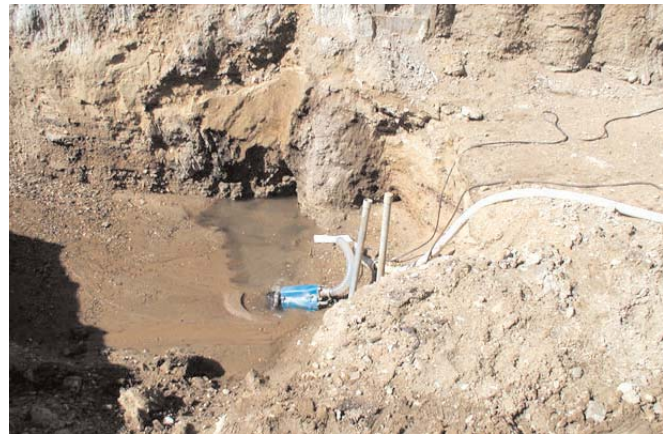
KTZ21.5 - horizontal, in on-shore-mode
