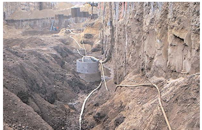
KTZ21.5 - dewatering by a drainage system
