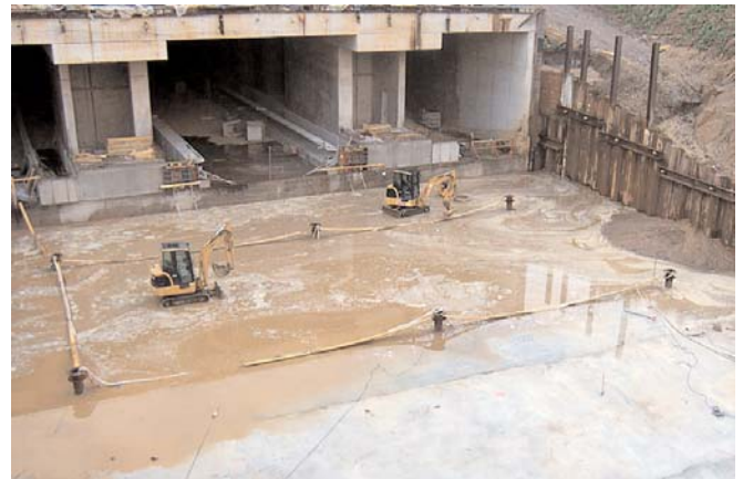
KTZ21.5 - well pots with submersible pumps
