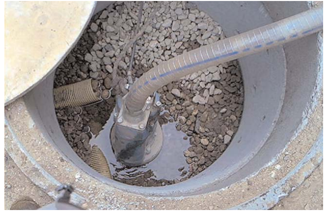
KTZ21.5 - installed in a drainage system to dewater the railway track
