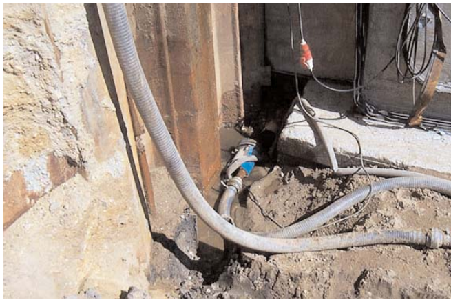
KTZ32.2 - dewatering in front of the existing tunnel entrance
