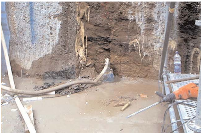
LB2-400 - minor dewatering when sealing the walls by means of small 1-phase submersible pump
